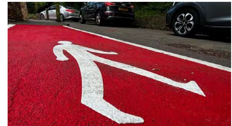
Figure 29. Example of a painted advisory sidewalk, an option for the 15th St bridge over Turkey Gully (Source: BBC)
