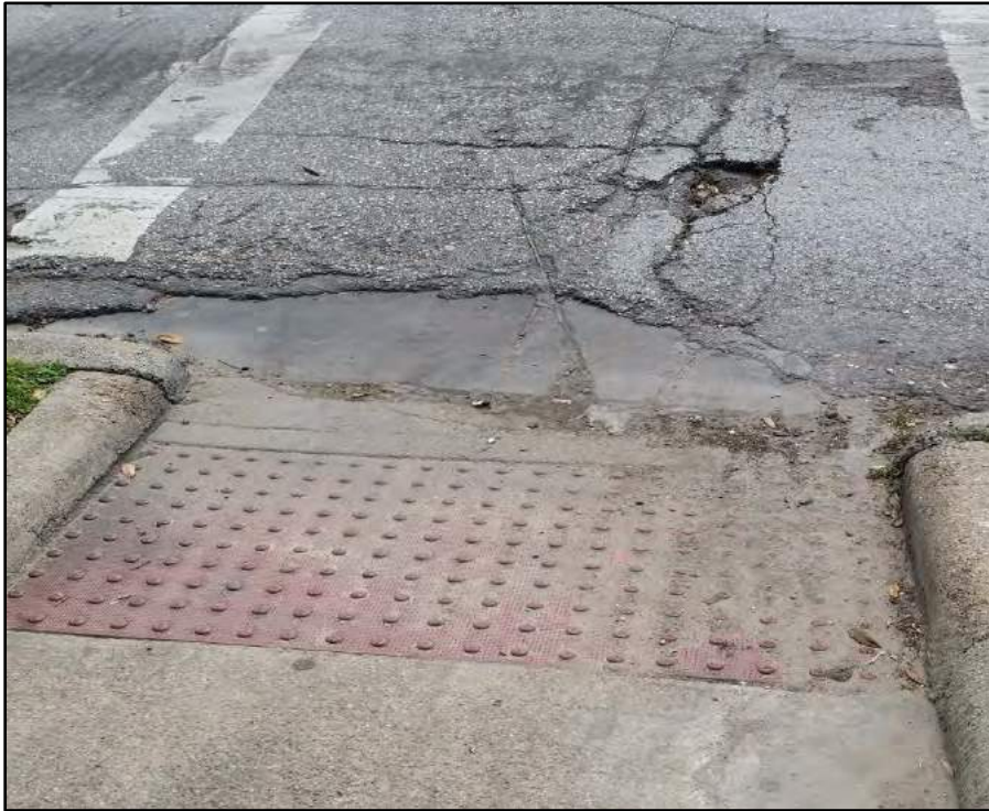
Photo 5 – Pavement Failure
