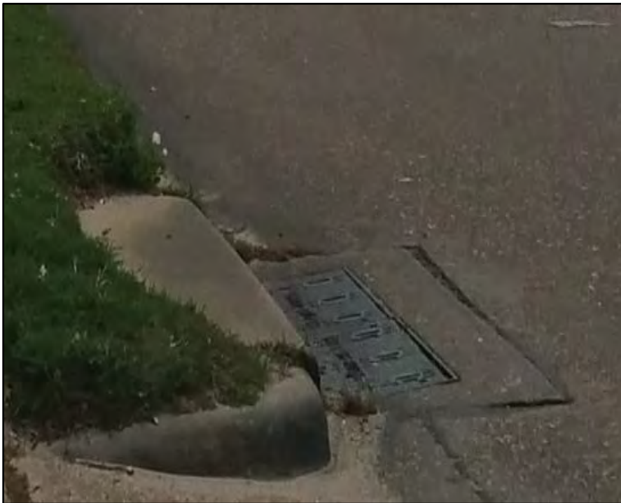
Photo 2 – Settling inlet
