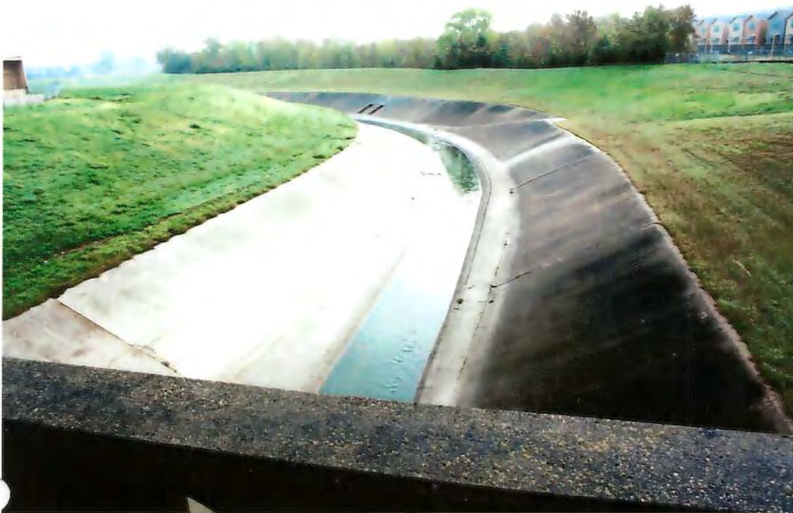
DOWNSTREAM VIEW FROM BRIDGE
