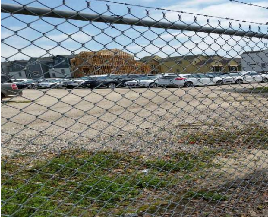
Photo 23 – Continued construction on Shepherd Drive
