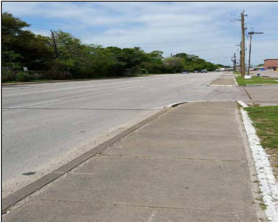
Photo 18 – Durham Drive behind Kroger
