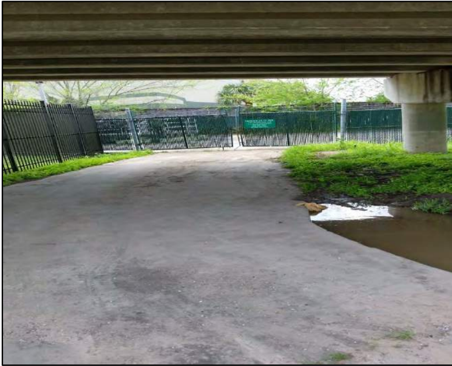
Photo 9 –Access Drive under Durham Bridge
