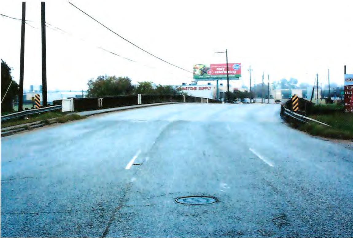
ROADWAY OVER BRIDGE
