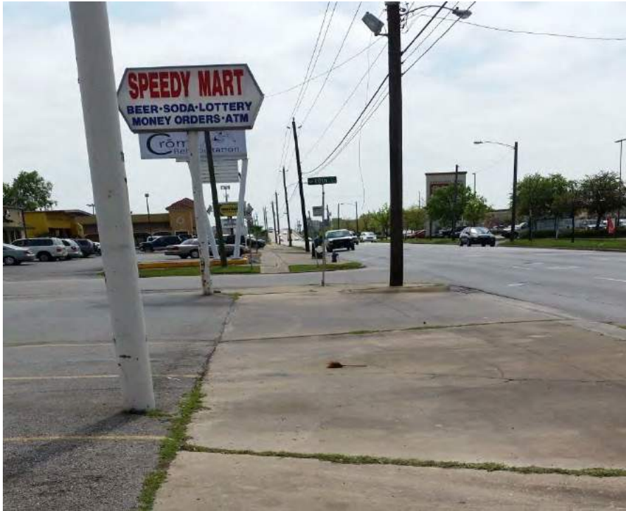
Photo 21 – Wider sidewalk that extends between the curb and right-of-way
