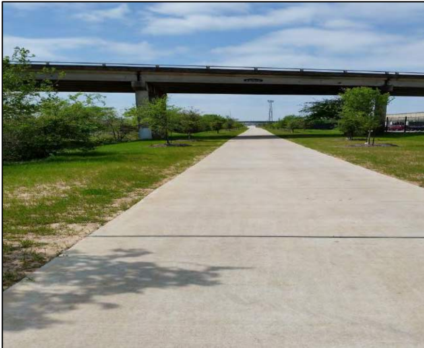
Photo 20 – Heights Trail west of Durham Bridge
