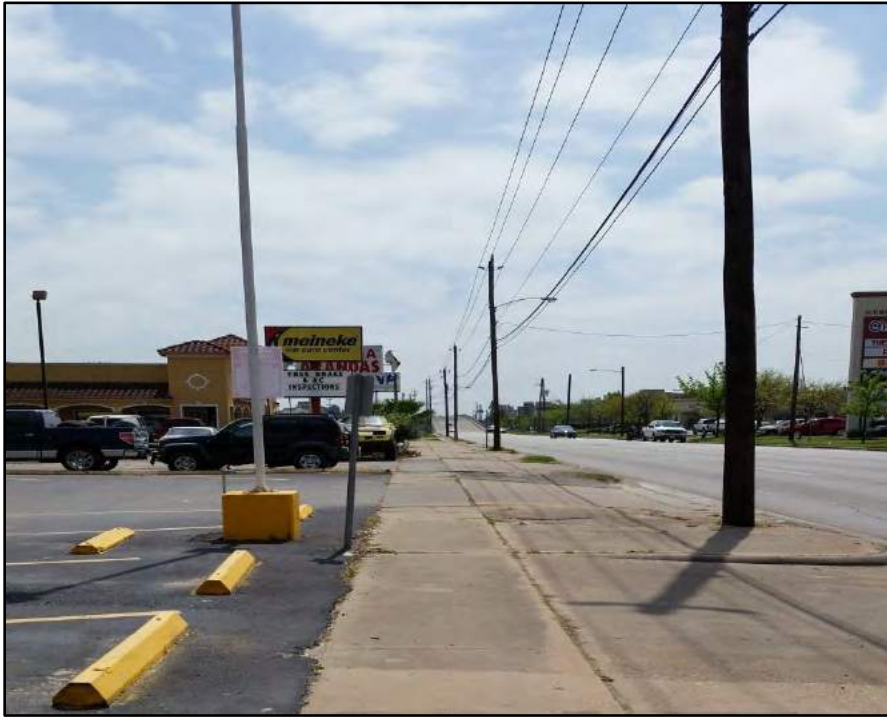
Photo 1 – Multiple driveways, grass growing in sidewalks
