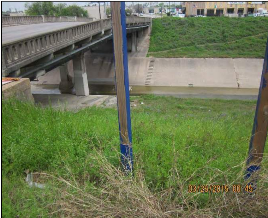
Photo 16 – Shepherd Bridge at White Oak Bayou
