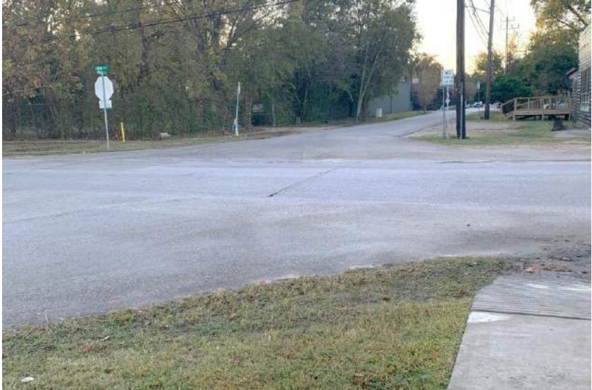
Figure 3. Existing Condition of the 19 th and Beall Intersection (Facing South)
