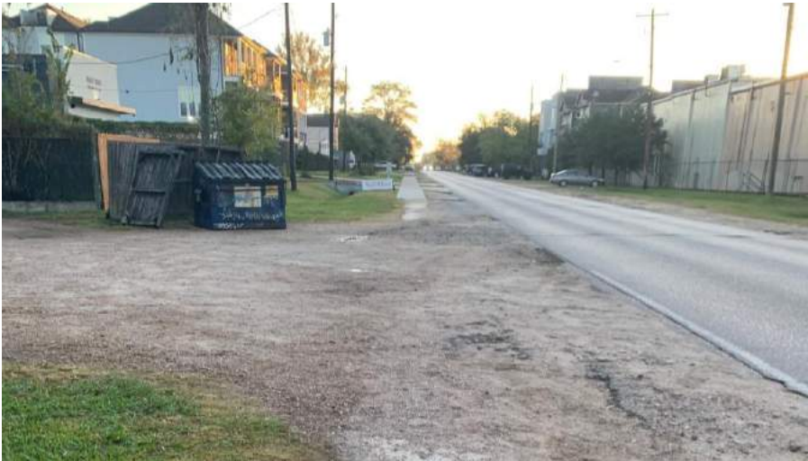
Figure 2. Current Sidewalk Condition along 19 th Street (Facing East)
